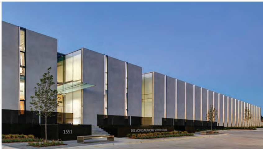
Figure 1. Des Moines Municipal Services, Neumann Monson
