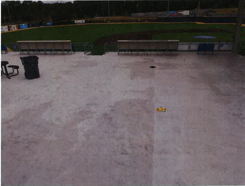
7. View Looking East at the Concourse Area Elevated Concrete Slab w/ Roof Canopy Steel Column K-4 (Right) in the Background.
