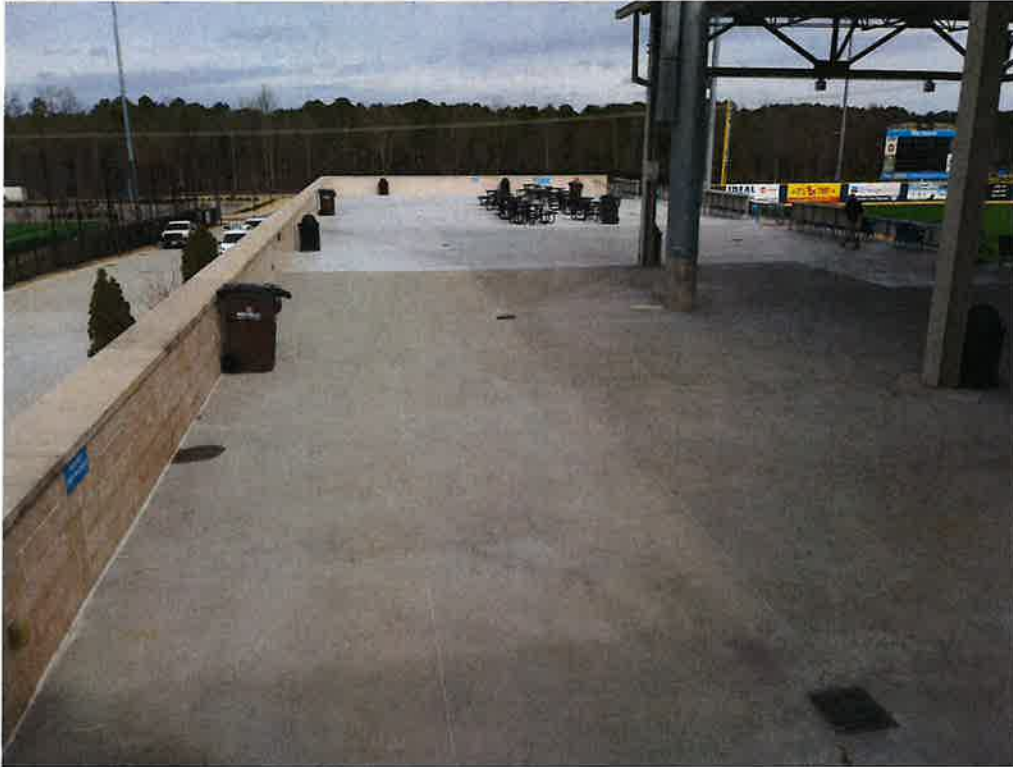
1. View Looking North Across the Concourse Area Behind 3 rd Base Line Along the Concrete Masonry Unit Parapet Wall (Left) at West Side of the Concourse.
