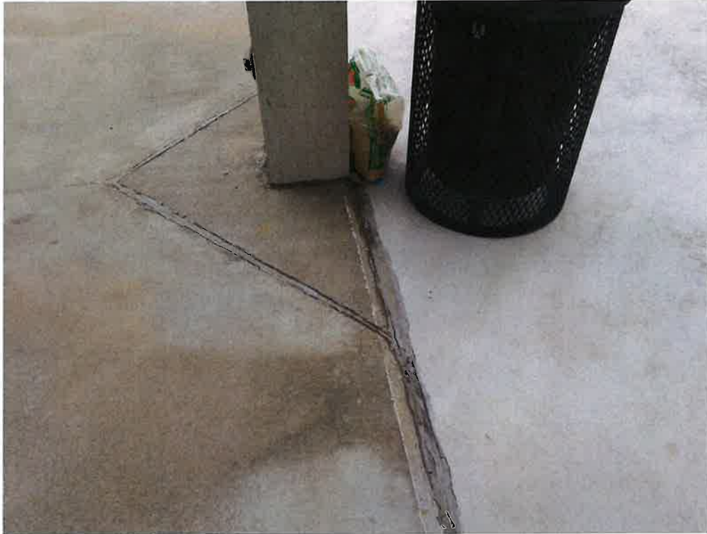
9. Close-Up View Looking at the Expansion Joint Assembly Between the Concourse Area Slab-On-Grade/Elevated Slab Assembly.
