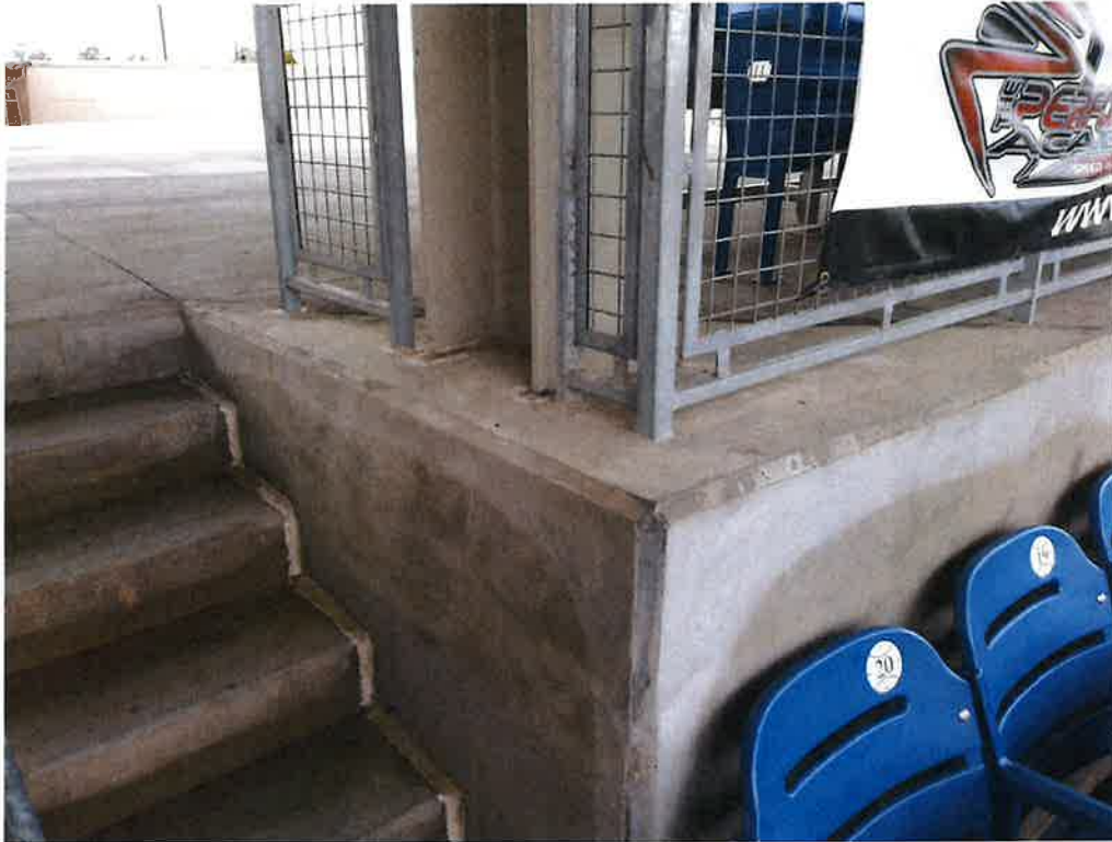
29. View Looking at Stadium Seating Area at the Exposed Corner Faces of the Slab-On-Grade at Column H-4.
