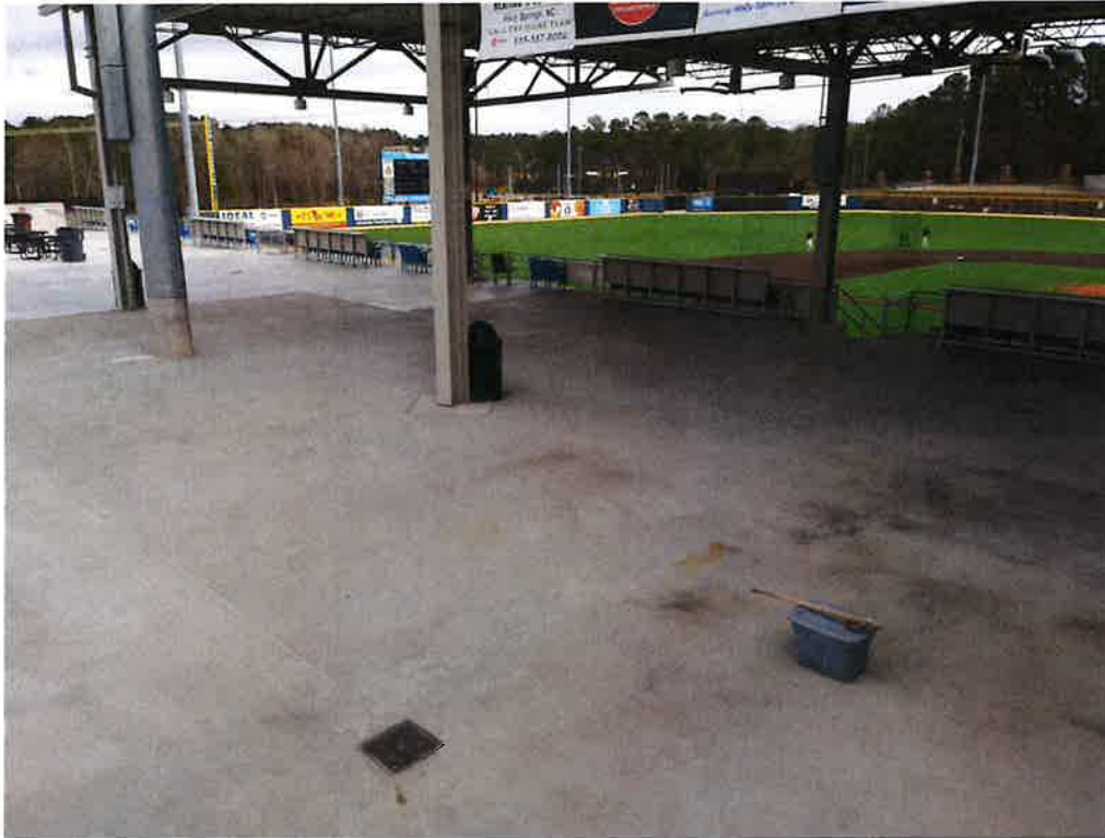
3. View Looking North East Across the Concourse Area Slab-On-Grade w/ Canopy Roof Steel Columns K-3 (Right), G-3 (Middle) & G-4 in Background.
