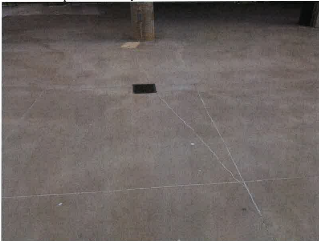
6. View Looking at Drain Assembly in the Concourse Area Slab-On-Grade & Control Joint Pattern.
