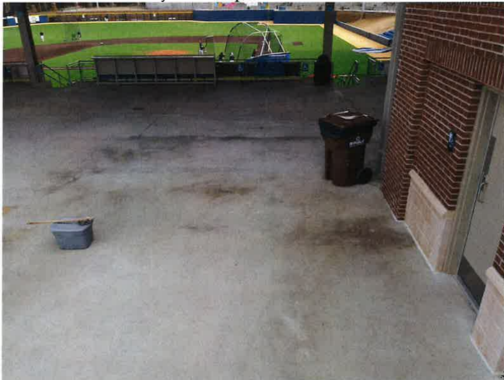
2. View Looking East at the Concourse Area Slab-On-Grade w/ Canopy Roof Steel Columns G-4 (Right) & H-4 in the Background.
