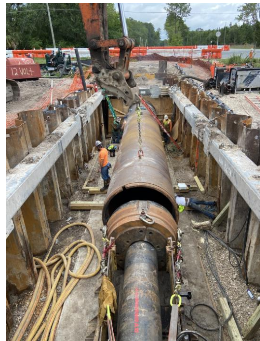
Figure 7-4: Pipe Ramming
