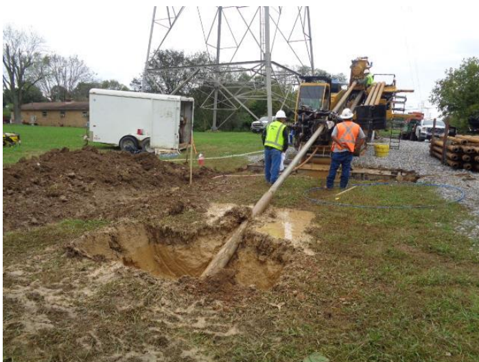
Figure 7-7: Horizontal Directional Drilling
