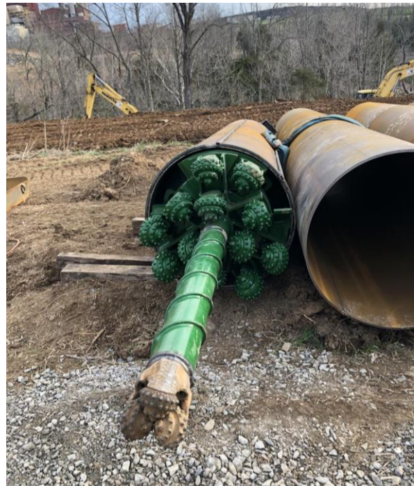
Figure 7-6: Pilot Tube Auger Boring
