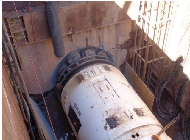
Figure 7-10: Tunnel Boring Machine
