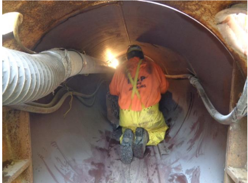
Figure 7-5: Pipe Jacking with Shield
