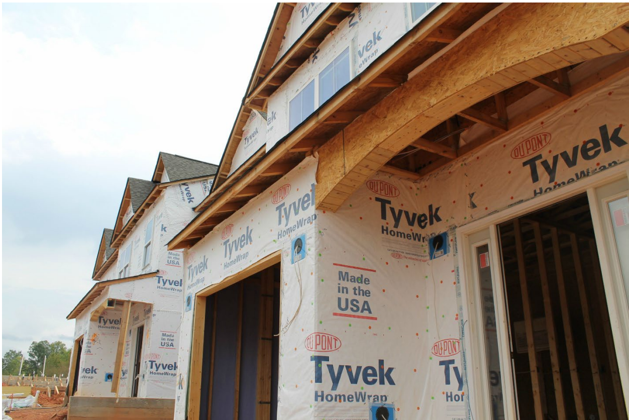
Image of townhome construction in Holly Springs
