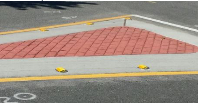
Typical stamped and colored concrete median hardscape. Brick pattern should be herringbone. For use Town-wide.
