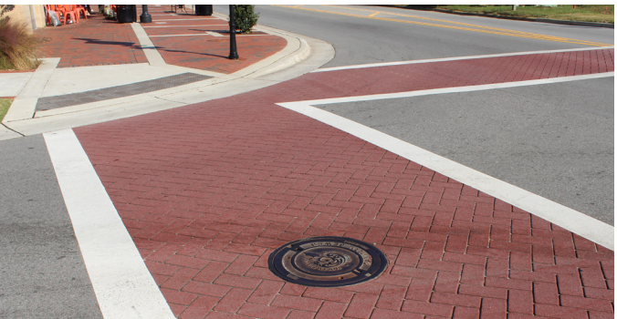
Crosswalks: Typical stamped and surface coat treated asphalt. Surface color applied with Endurablend or equal product. For use town-wide and Downtown Village District
