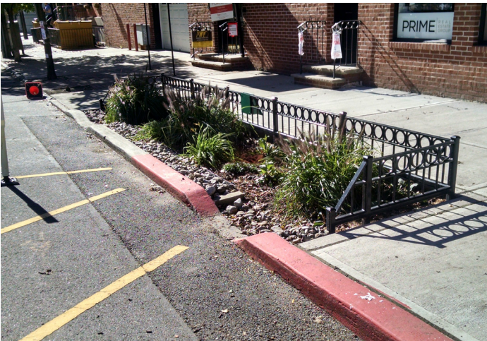
Example of stormwater bio-swale.
