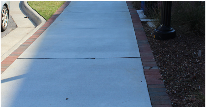
Typical concrete sidewalk with single brick soldier course border; Downtown Village District Area use only. No brick soldier course border for town-wide use.
