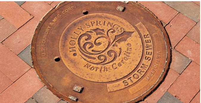
Typical custom manhole cover within sidewalk; Downtown Village District use only. Non-custom covers for town-wide use.
