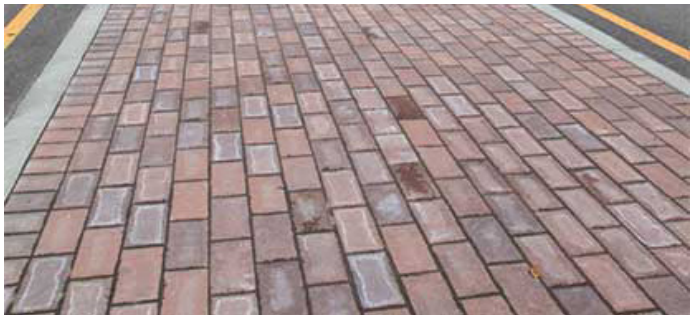
Example of paver hardscape median with running bond pattern and single soldier course border for use within Downtown Village District. Pavers should match sidewalk pavers.
