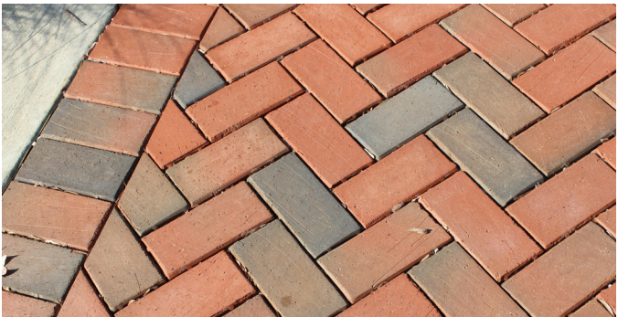
Typical permeable brick paver in herringbone pattern and single soldier edge course in furnishing zone of streetscape; Downtown Village District Area use only.
