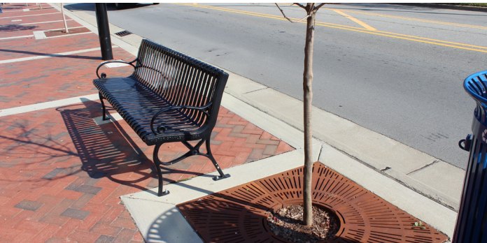
Example of existing bench and tree grate along S. Main Street, Holly Springs. Benches should be mounted on concrete pads as shown.
