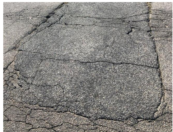
HIGH Severity Patch
