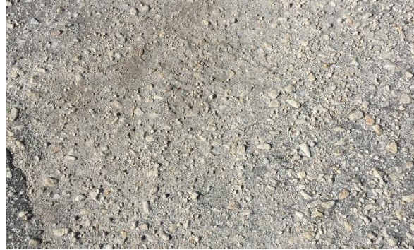
HIGH Severity SD
