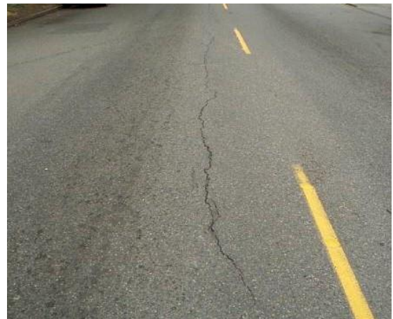
LOW Severity FC
