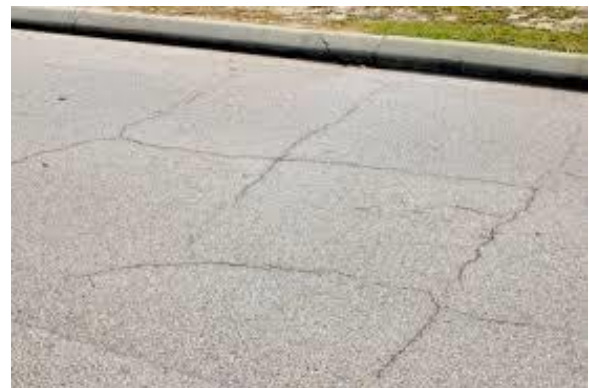
LOW Severity BC
