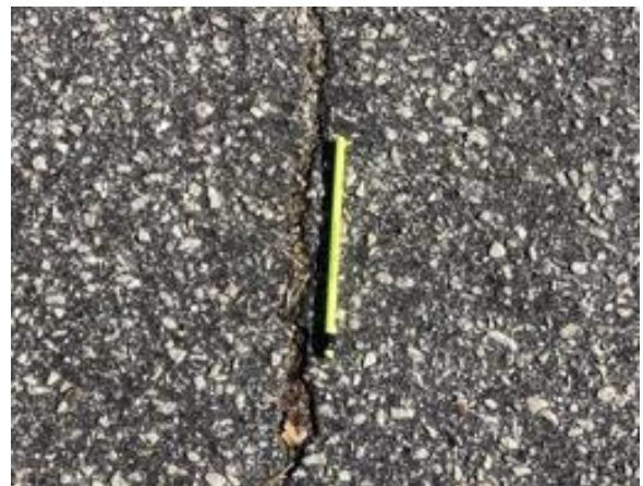
MEDIUM Severity TC
