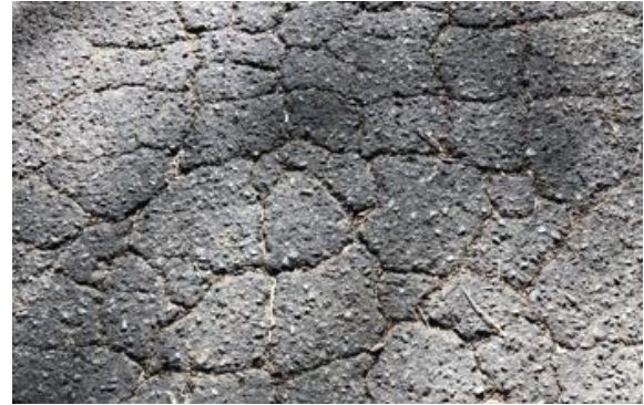
HIGH Severity FC
