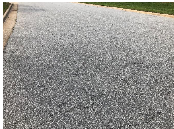
MEDIUM Severity BC
