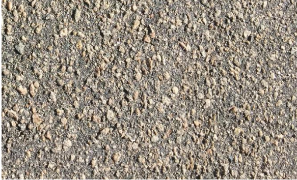
MEDIUM Severity SD
