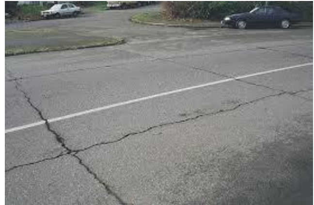
Reflective Cracking
