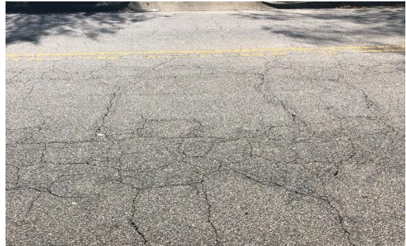
HIGH Severity BC
