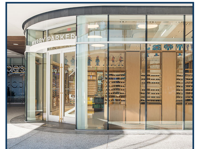
Curved facades create contrast in shape
