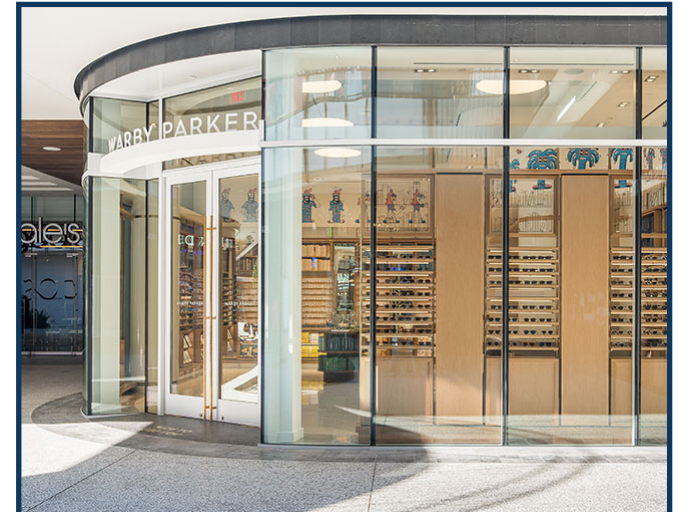
Curved facades create contrast in shape
