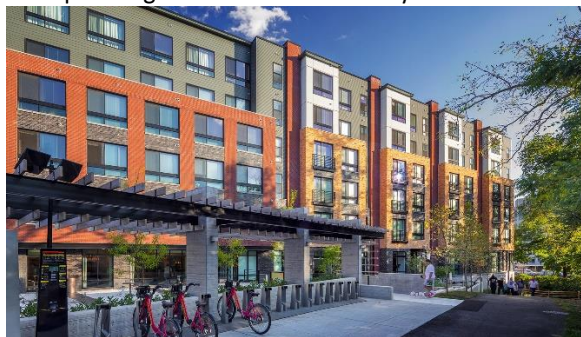
Example Image – Mid-rise multifamily residential
