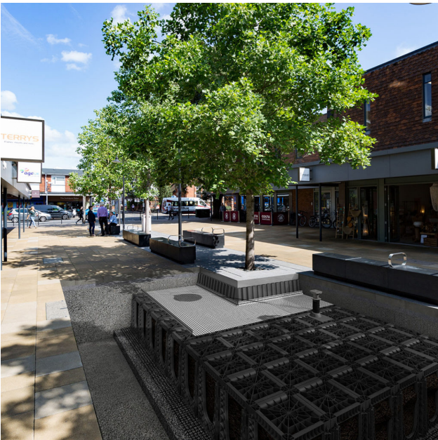
Soil cells allow tree roots to extend beyond the planting zone by supporting uncompacted, nutrient-rich soil within a 3-dimensional structural grid. (Image courtesy GreenBlue Urban)
