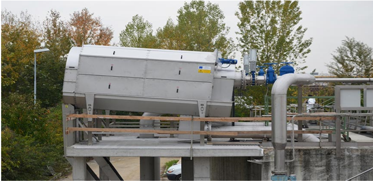
Figure 2-5: Rotary Drum Screen
