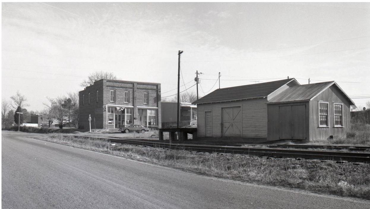
Second depot of Holly Springs after the first one burned down. Seagraves Drugstore in background. Signal Maintainer Roy Wilson's motor car shed (see The Railroad Press article).
