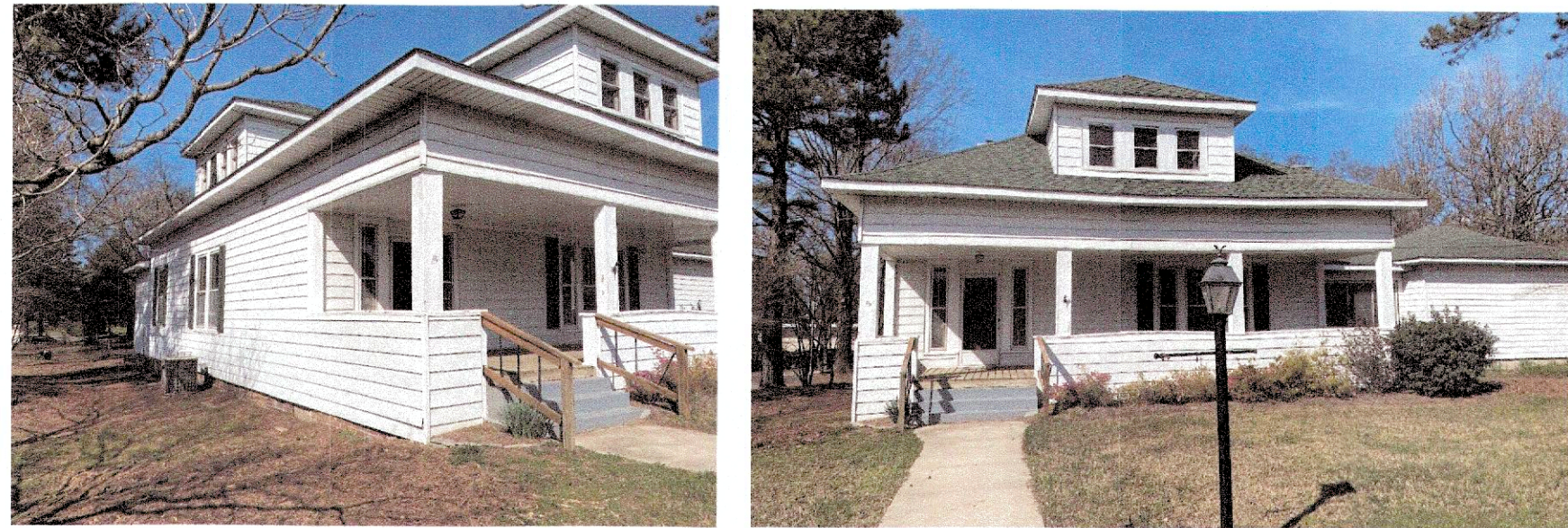
WEST FACING - SIDE EXTERIOR SOUTH FACING - FRONT EXTERIOR
