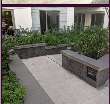
Green Stormwater Devices mitigate runoff
